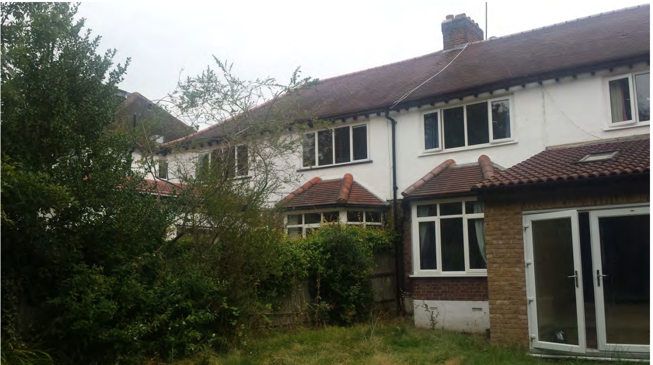
Rear towards no. 2 Canons Close
