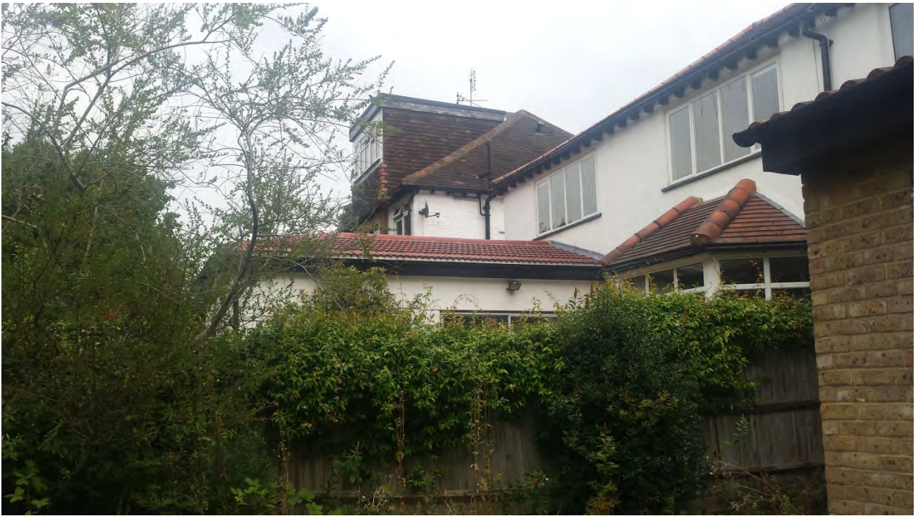
Single storey rear extension at no. 2 Canons Close
